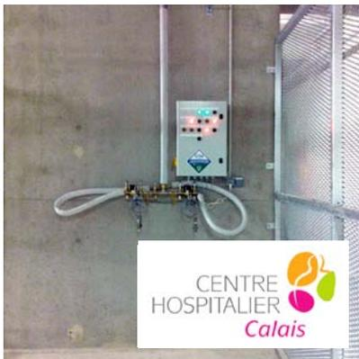
In cooperation with Dohmeyer NV of Belgium Cryo Solutions has installed a switch over device for pressure tanks in the service basement of the Hospital in Calais France. From this unit, vacuum insulated piping runs up to the IVF centre in the second floor where - cryopreservation takes places.
